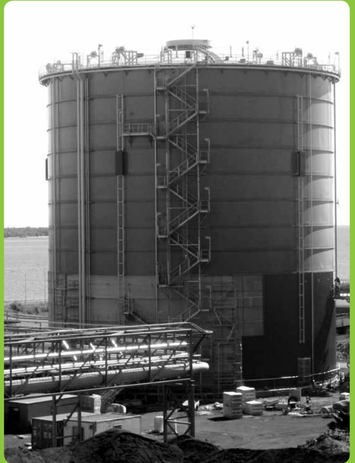
The carbon monoxide gasholder in Tornio.
